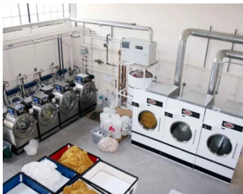
MACHINE SERVICING & MAINTENANCE
